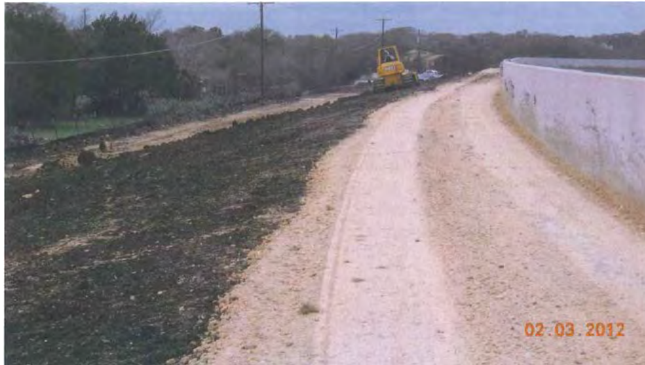
Repair of slope failure caused by Tropical Storm Hermine at Dam 13A
