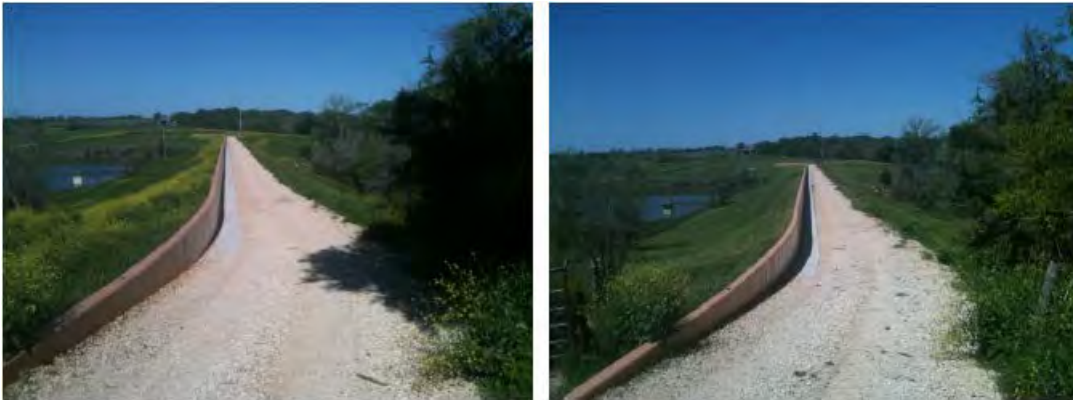
Dam Maintenance at Dam 21 – Before and After
