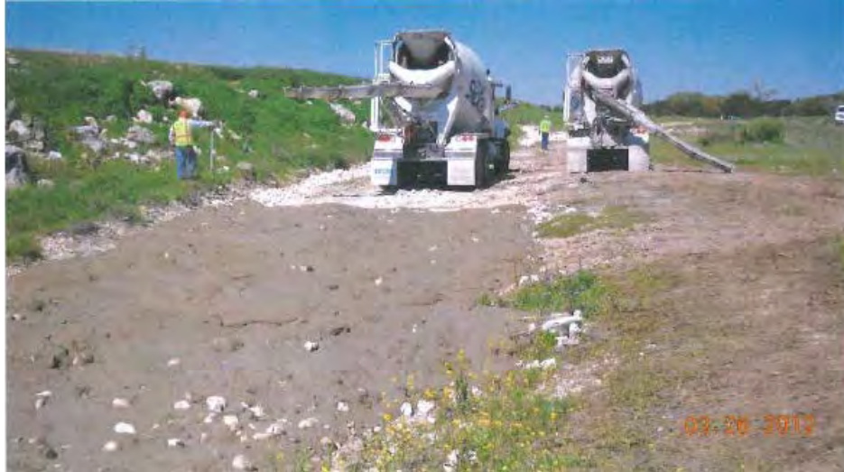
Repair of Erosion caused by Tropical Storm Hermine at Dam 6 Auxiliary Spillway
