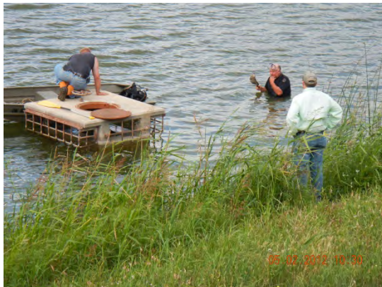
Old Drain Valve being removed at Dam 20
