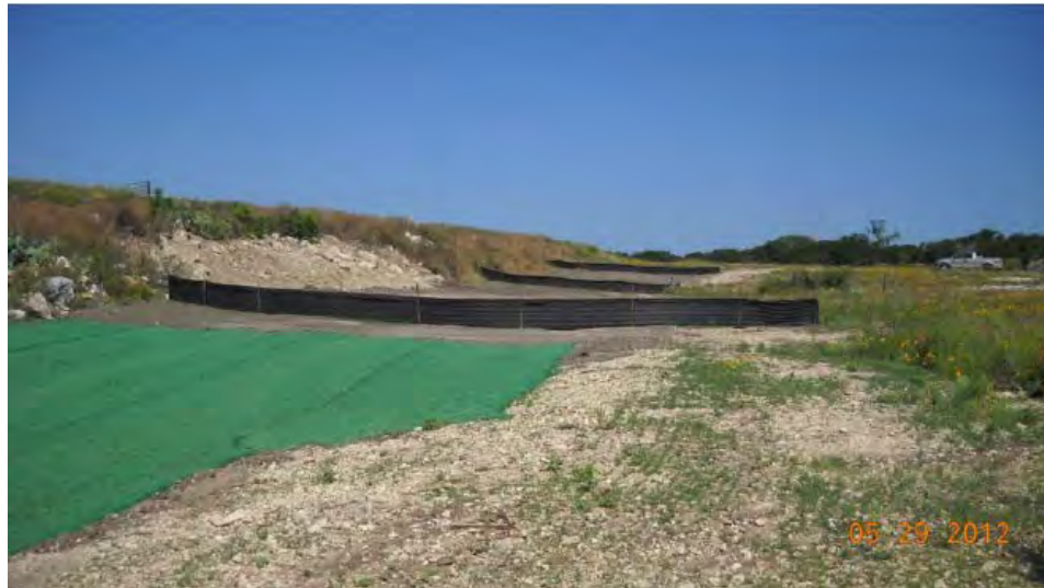
Repair of Erosion caused by Tropical Storm Hermine at Dam 6 Auxiliary Spillway
